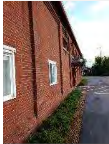
Photo 15 – Non-asbestos brick mortar at the perimeter of the building.
