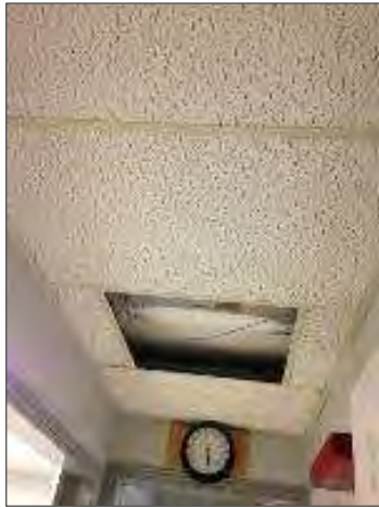
Photo 7 – Non-asbestos 24" x 48" lay-in acoustic ceiling tiles in the 2 nd level kitchenette.
