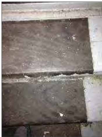
Photo 12 – Non-asbestos stair tread on the basement stairs.
