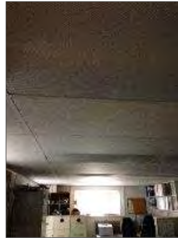
Photo 8 – Non-asbestos 24" x 48" lay-in acoustic ceiling tiles in the main floor office.
