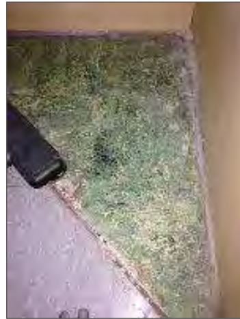
Photo 10 – Non-asbestos 9" x 9" vinyl floor tiles in the 2 nd level classroom area.
