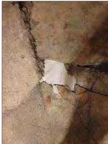
Photo 11 – Non-asbestos levelling compound in the basement.
