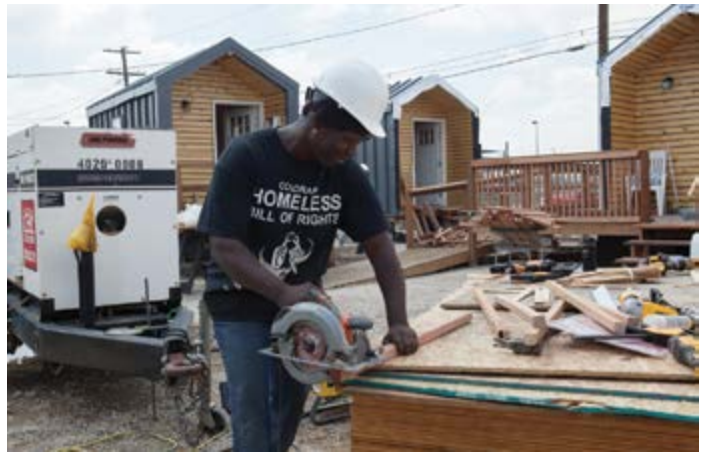
Construction at the village. Image credit: JC Buck
