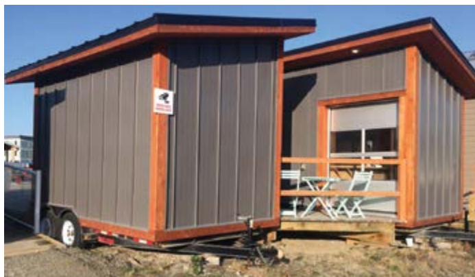
Moveable tiny house used as a business in Carcross, Yukon. Wheels remain on the unit and a boardwalk is built around it so they aren't visible at first glance
