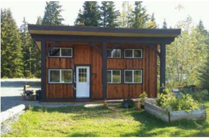
Entrance of a tiny house in the community. Image credit: Bluegrass Micro Village
