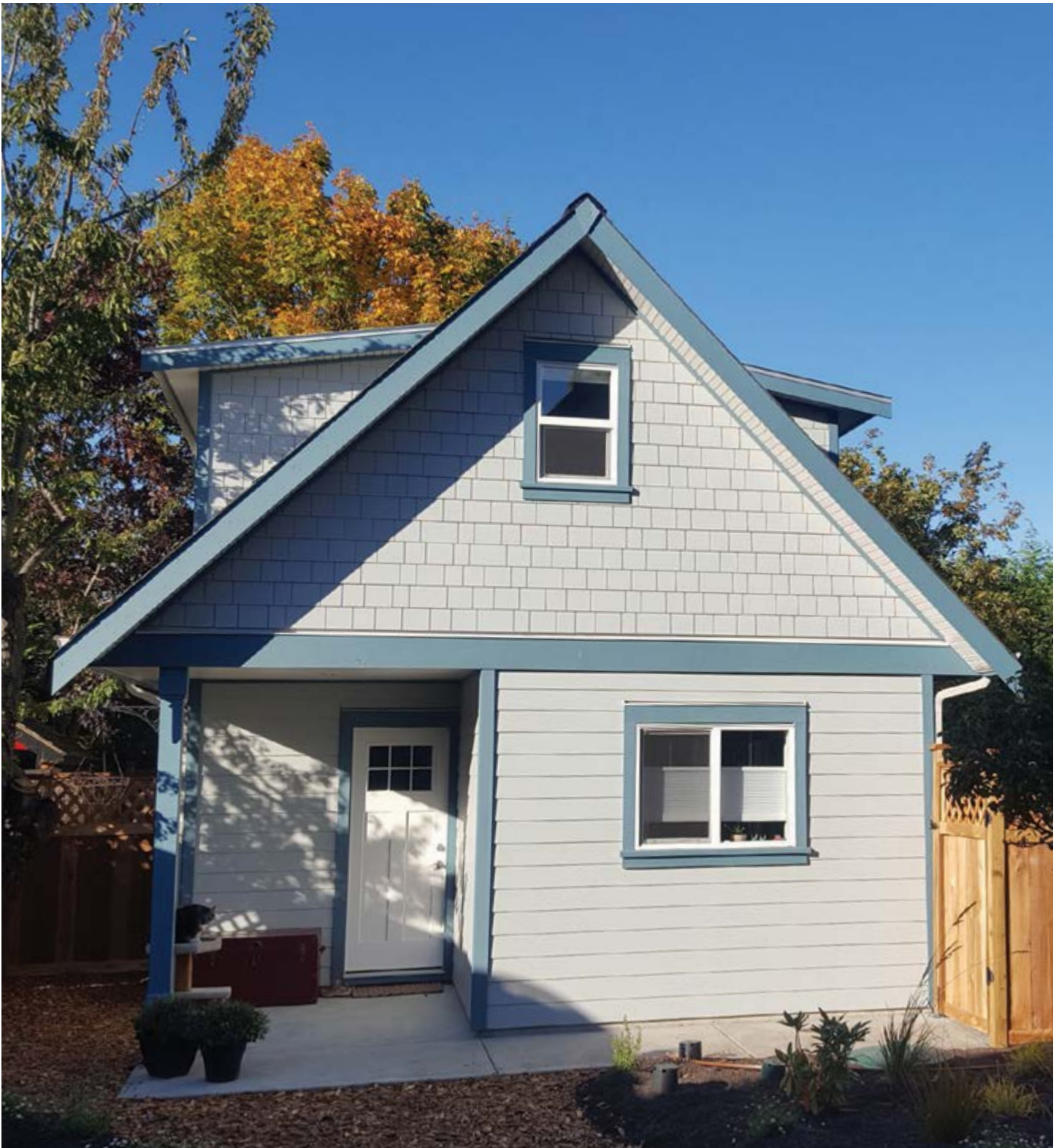
A garden suite in Victoria. Image credit: City of Victoria
